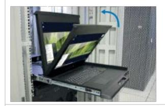
Step 2 Flip up the LCD to a suitable viewing angle
